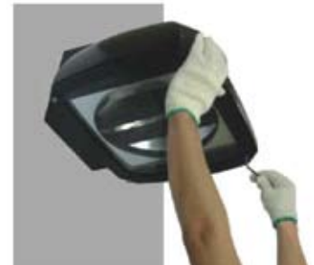
1. Level bracket and install on wall.
